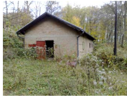
Figure 7 Another warehouse on Horvati site
